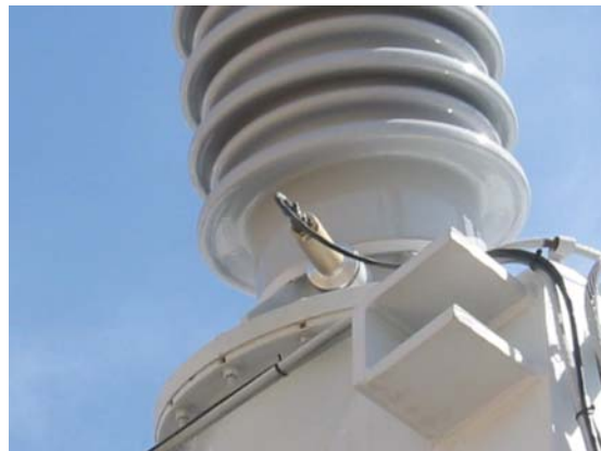
Figure 6 - Typical In service BTC connection
